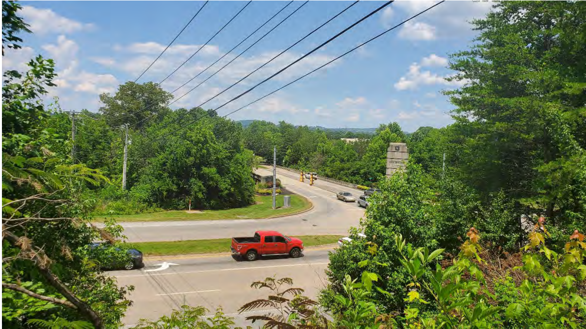
Photograph 9: View of electrical transmission line crossing Hardin Valley Road from the northern subject property boundary.
