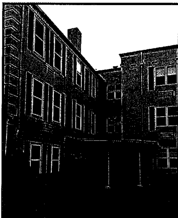
RIVER OAKS PLACE, LOUDON TENN.
