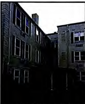
RIVER OAKS PLACE, LOUDON TENN.
